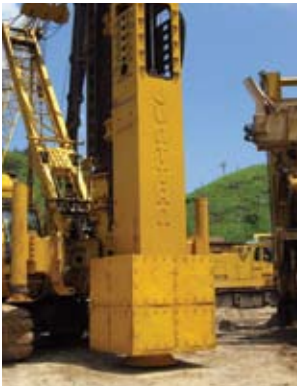
Acoustic enclosures for piling hydraulic hammers cut noise pollution significantly and reduce disturbance to local communities.
