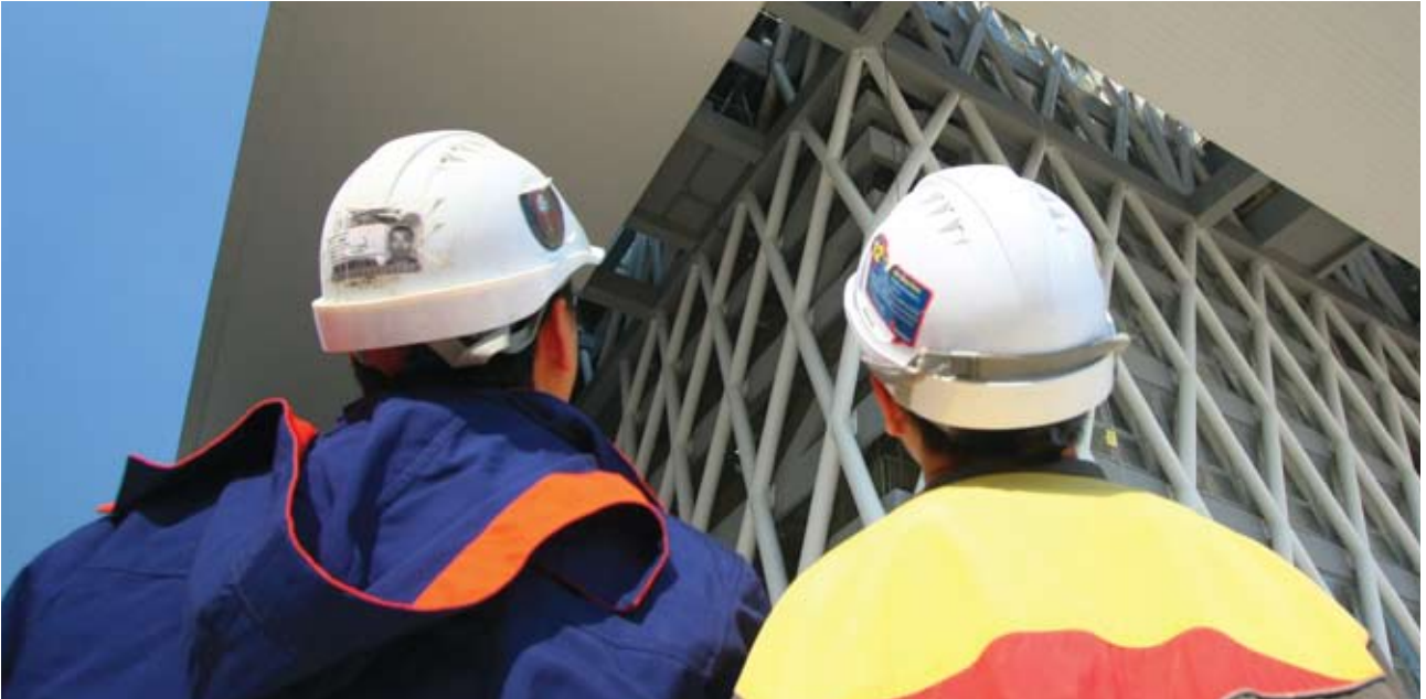
Structural steelwork for new campus of Vocational Training Council, Hong Kong.
