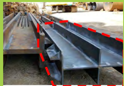
Reusing stanchion followers on the Murray Road foundations project to reduce the need for 50 tonnes of steel plate.
